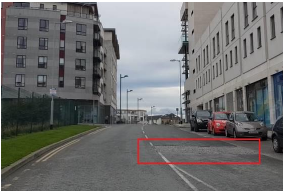
Figure 8: Unfinished carriageway on Station Street
