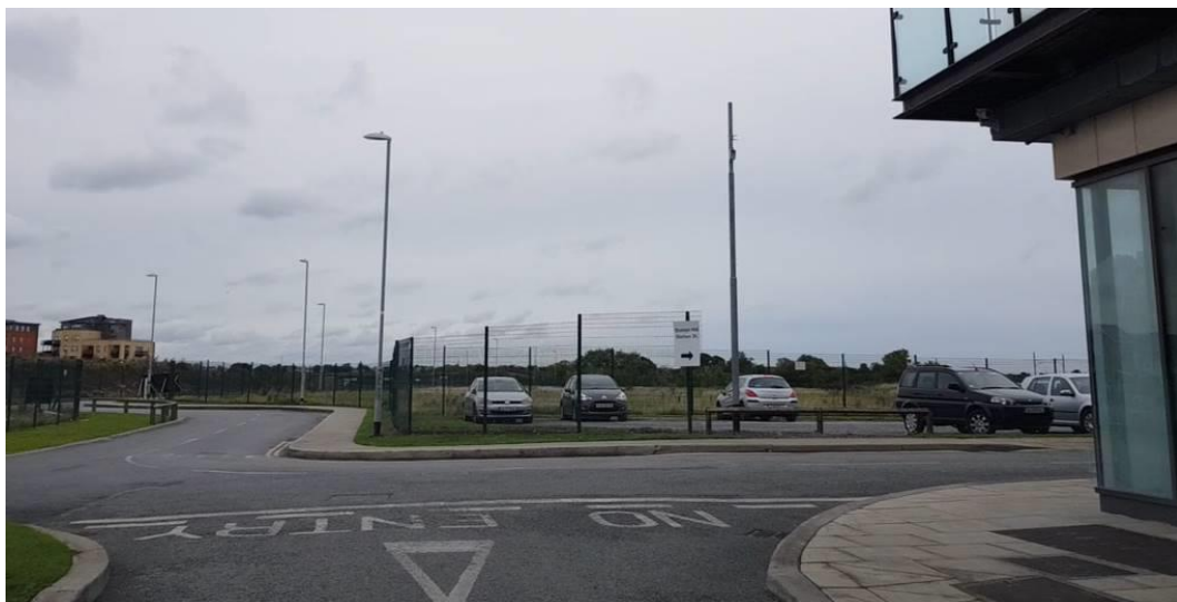
Figure 18: Building Line restricting forward visibility at Yield Control
