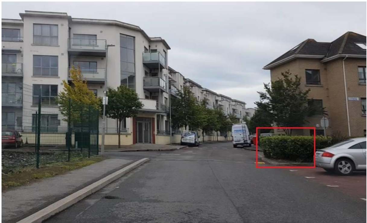
Figure 13: Landscaping presenting an obstruction in junction visibility splay
