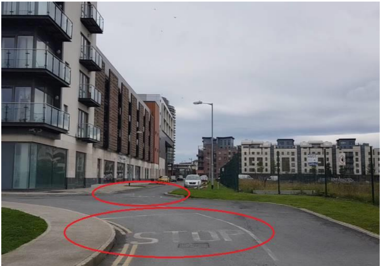
Figure 25: Ambiguous Form of Control at Existing Junction
