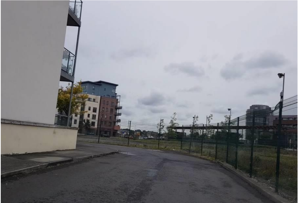
Figure 16: Building Line restricting forward visibility on Dargan Lane
